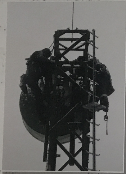
MONTAGE STATION GÖSSKAR
